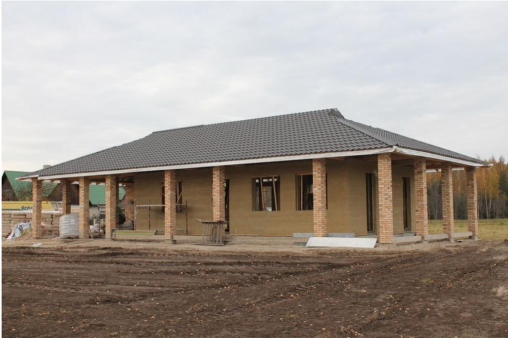
*Figure 1. HEMP ECO SYSTEMS LATVIA hemp building, in-situ method.*
